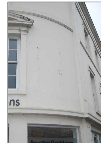
Schedule of Dilapidation's Ref No. 4 Clause No 5.4 Fill and repair old fixing holes to external walls over ground floor shop entrance ready for redecoration
