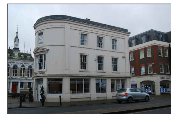
Schedule of Dilapidation's Ref No. 1 and 2 Clause No 5.23 and 5th Schedule, and Clause 5.4
