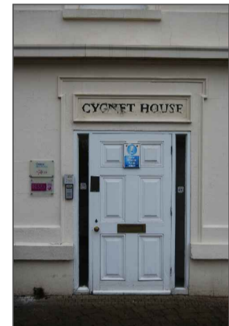
Schedule of Dilapidation's Ref No. 6 Clause No 5.4 Remove sign over ground floor office entrance and provide new stainless steel entrance sign over the door - see D&A statement for example of new sign Schedule of Dilapidation's Ref No. 7 Clause No 5.5.2 Remove sign to left hand side of ground floor office entrance. Fill/repair holes ready for redecoration. Provide new signage to clients approval
